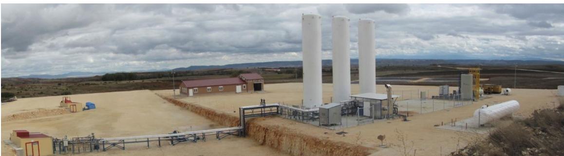
CIUDEN Hontomín plant in Spain will be hosting the course on monitoring large scale CCS pilot R&D facilities.
