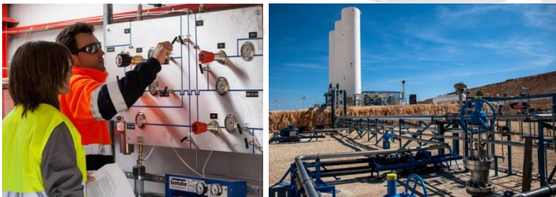
Operation at one of the ECCSEL Research Infrastructures. CO 2 Storage Development Plant located in Hontomin (Spain).
